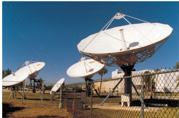
Lightning Protection on Dishes
